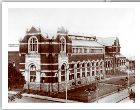
Hackett Hall viewed from James Street with the Jubilee Building in the background.
