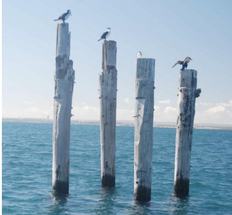
Figure 5: Timber pile structure off Garden Island since identified as Dolphin No. 60 in April 2007 after loss of timber platform bracing in a storm in 2006, view looking southeast. (Patrick Baker / WA Museum)
