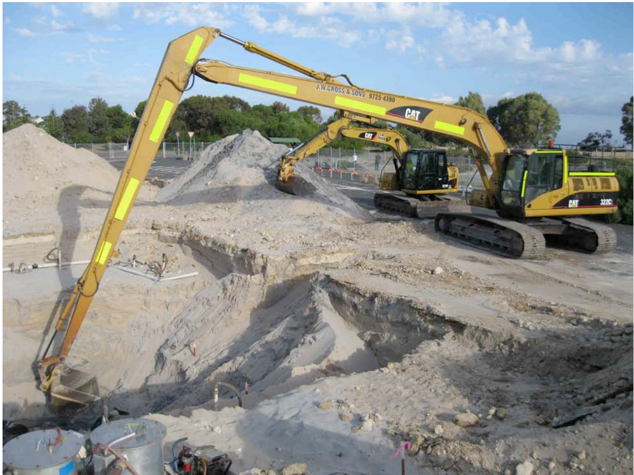
Figure 27. Long and short arm excavators on site (Ross Anderson/ WA Museum).
