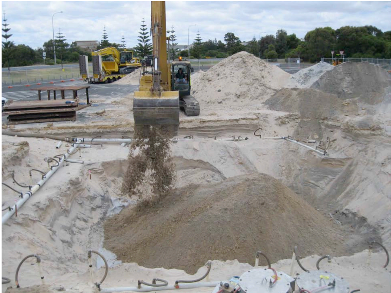
Figure 51. Backfilling Lot 882 Trench 1 over layer of geo-textile (Ross Anderson/ WA Museum).
