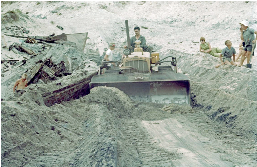
Figure 5. Bunbury shipwreck Site K/ North America (1843) being exposed by Cable Sands Company bulldozer operator Mr Leo Sophilis (WA Museum).
