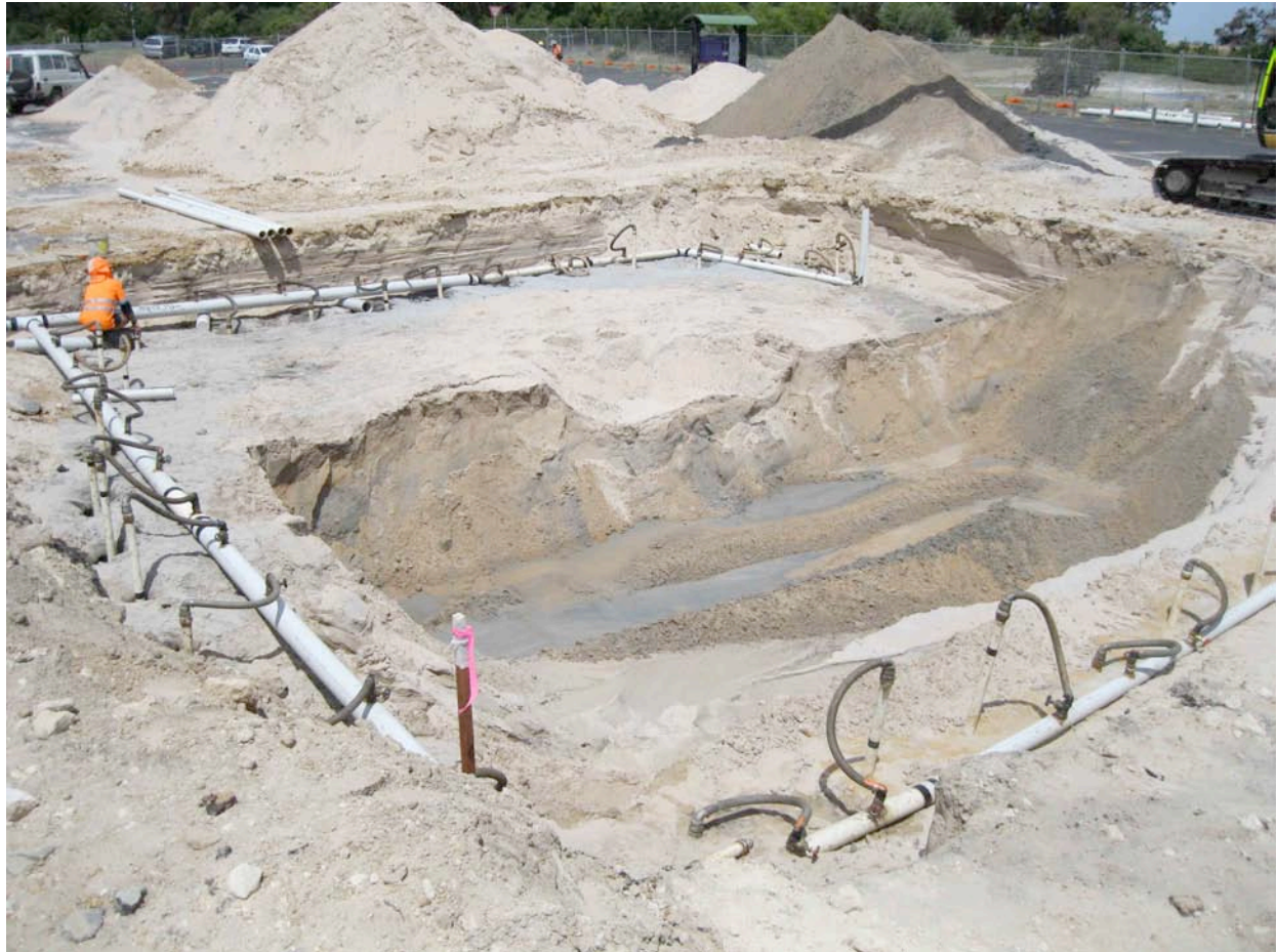
Figure 26. Dewatering system being installed on Lot 882, view north (Ross Anderson/ WA Museum).
