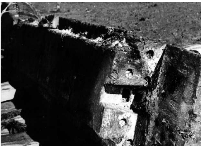
Figure 77. Photograph of keel scarf at the time of excavation showing the baosongkong .
