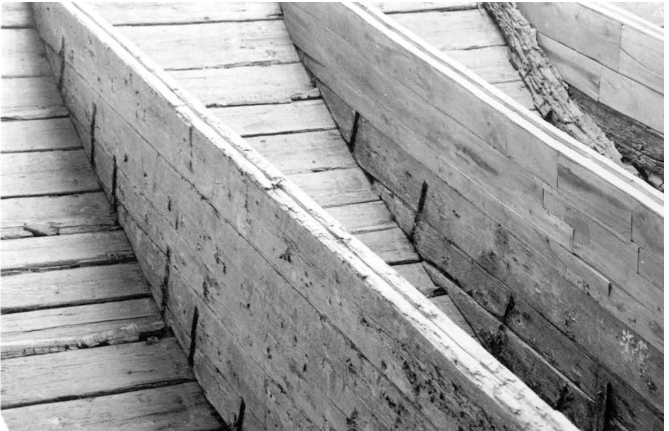
Figure 85. Photograph showing the bulkheads 4 to 9 (right to left) just aft of the mast step with the stiffeners (note to the right, the bulkhead with the frame on the aft side).
