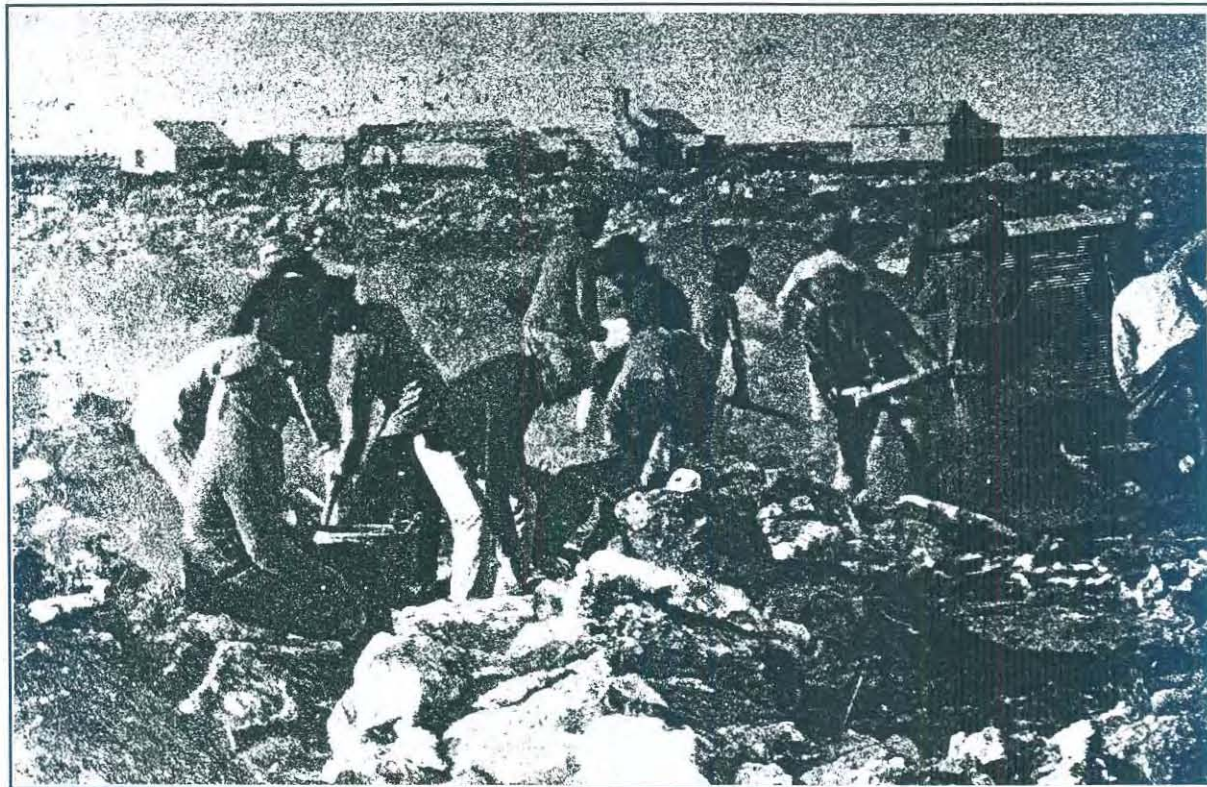
Figure 24. Guano miners at work on Rat Island with settlement buildings in the background to the north-east (photo: W. Saville-Kent coll. BL 1786B/13).
