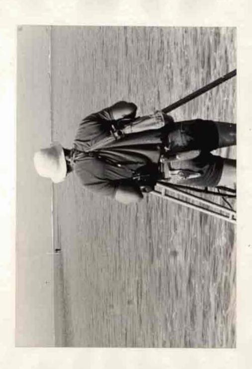
Fig. 6. Setting up the theodolite on the reef to eventually take readings of the buoys on the wreck site.
