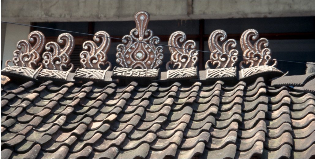
Figure 197: Ridge tiles from the Kudus—Jepara area are used by an antique shop in Ciputat Raya in Jakarta, as decoration over the roofed entrance to its premises.
