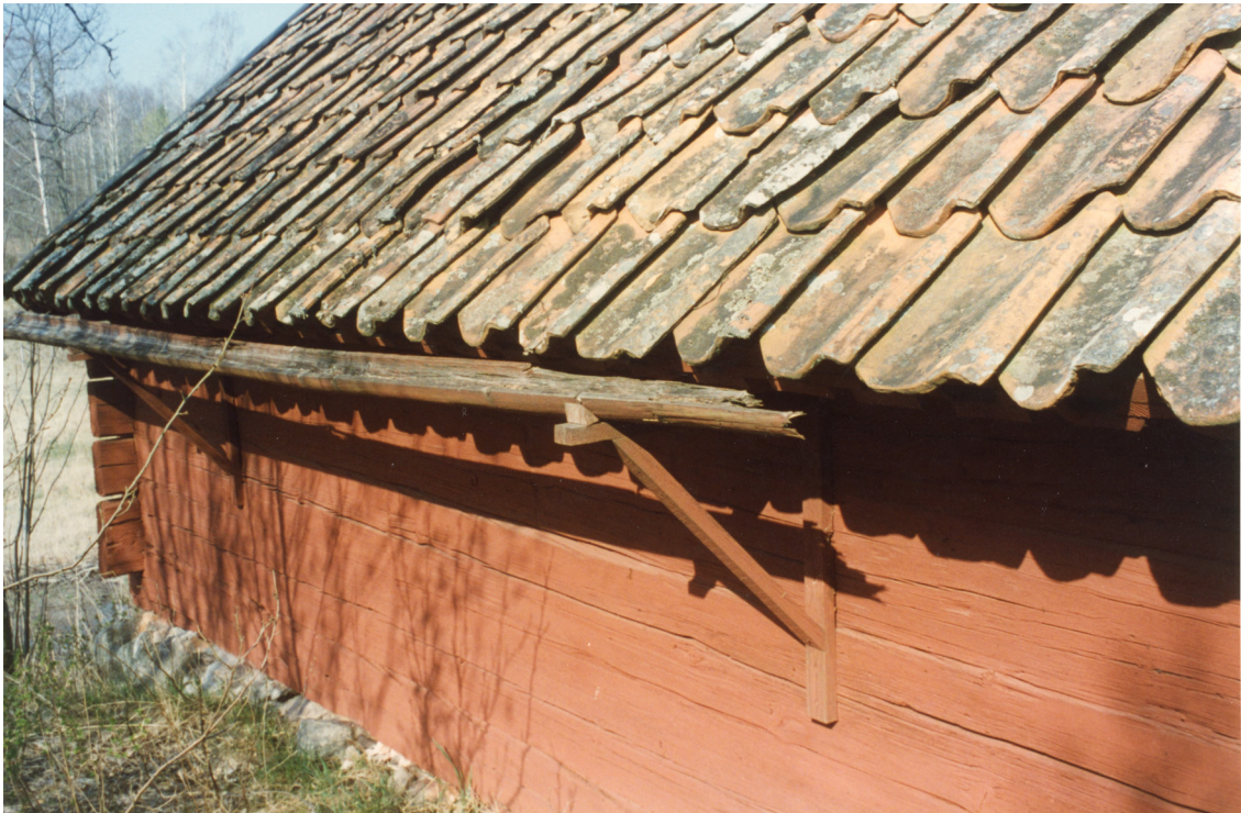
Figure 184B: Old cellar roof in Sweden covered by the Dutch type of roofing tiles.
