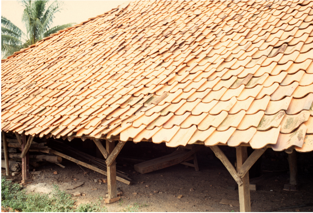
Figure 184A: Tiles covering a brickworks roof at Bekasi, West Java.
