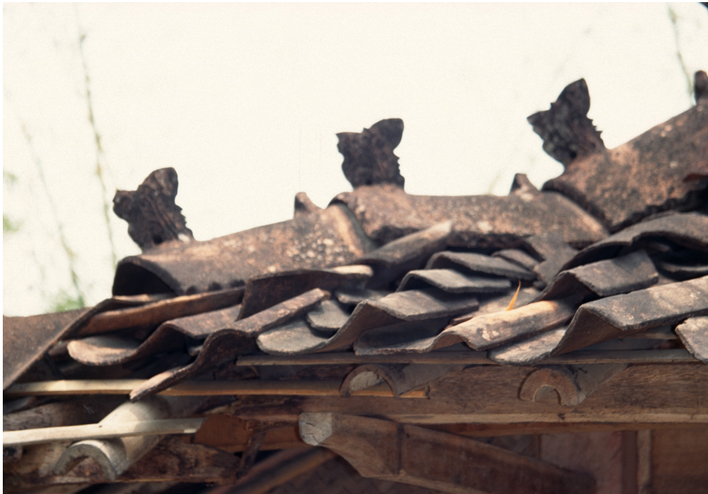
Figure 200: Hip tiles and pan tiles on a roof, Kudus area.
