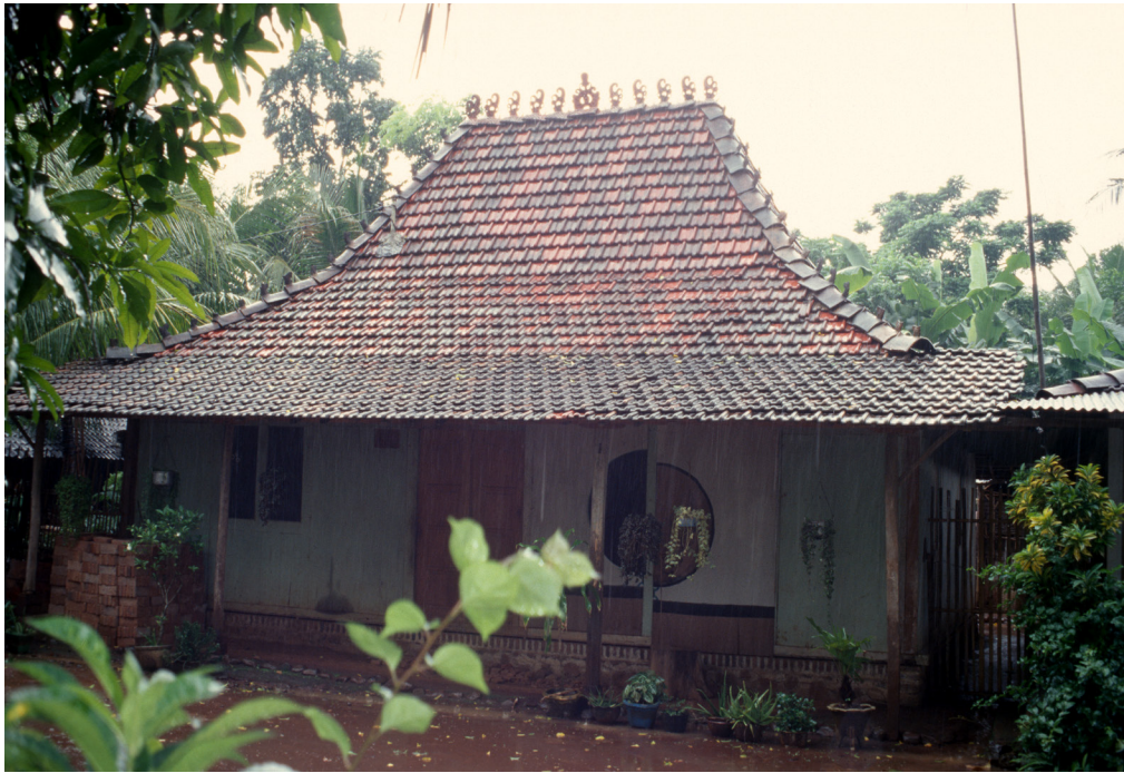
Figure 193: Rumah limasan , house with a four-section pyramidal roof, in Bandung Indah, close to Bangsri, Central Java, with decorated ridge tiles, genteng kelir .
