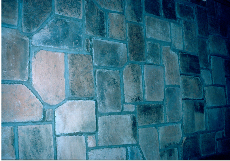
Figure 175: Wall made of Majapahit (possibly paving) bricks.
