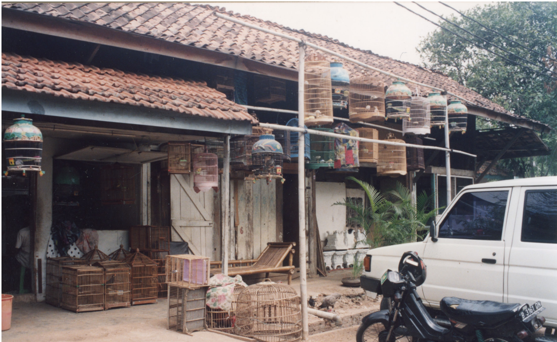
Figure 177: House in Jakarta covered by two types of commonly used roof tiles.
