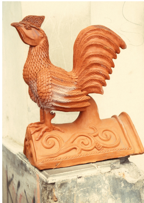
Figure 192: Modern Wuwung jago , rooster ridge tile.
