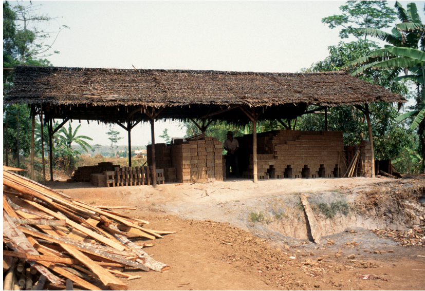
Figure 167: Brick kiln, tombong bata , under protective, removable thatched roof at Désa Kali Manggis, Kecamatan Subah, Kabupaten Dati II Batang, Central Java.
