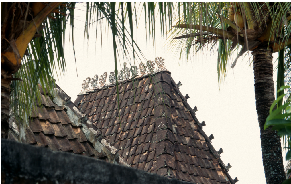
Figure 194: Steep upper section of joglo house with ridge tiles, and a row of cockscorn hip tiles, bandongan .
