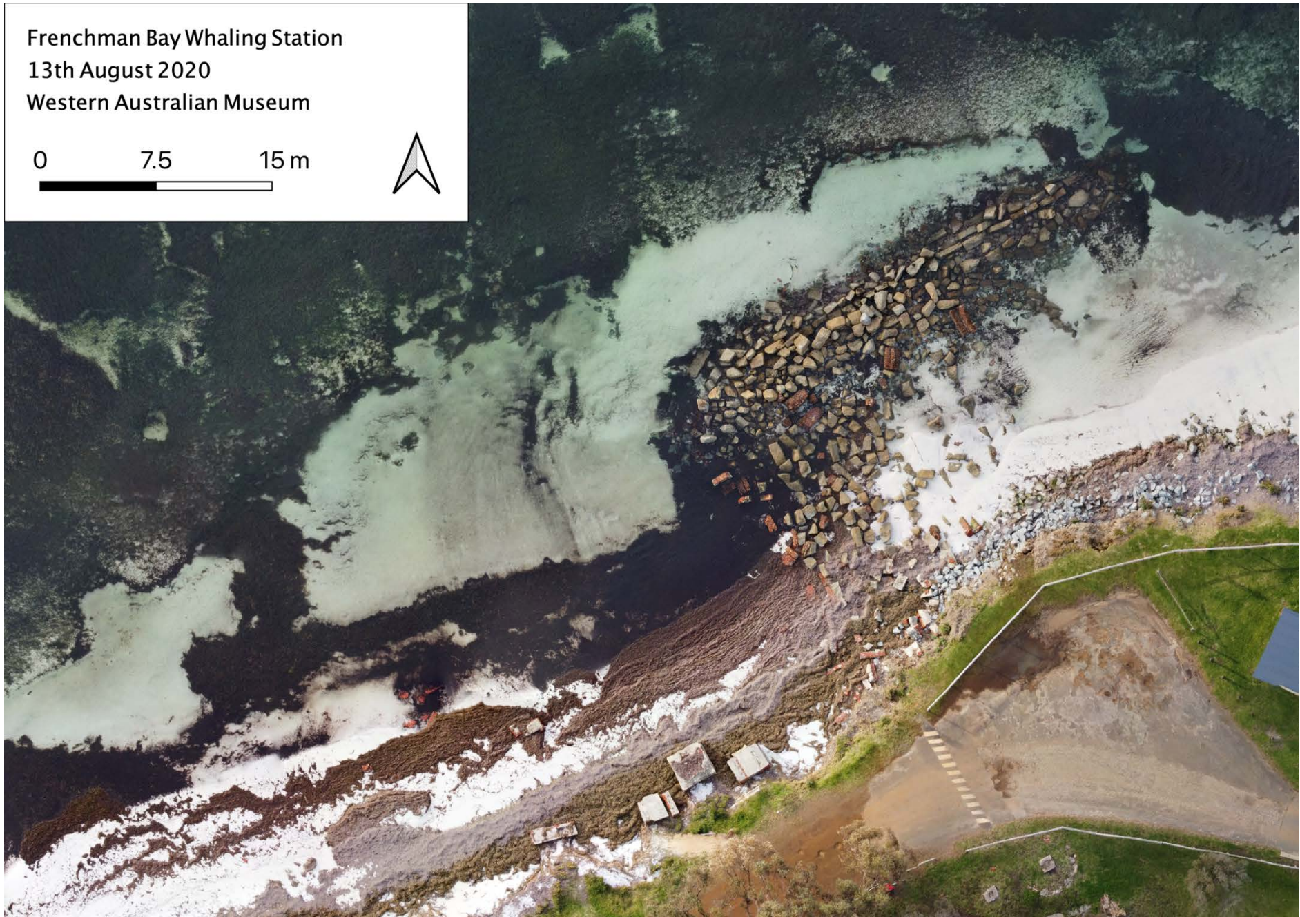
Figure 12. Frenchman Bay Whaling Station orthomosaic. Recorded by Mavic Mini drone and processed in Agisoft Metashape. (Patrick Morrison/ WA Museum).
