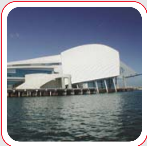
The new Western Australian Maritime Museum.
