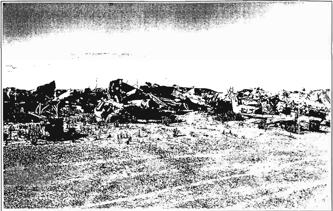
Figure 9. Material from Town Jetty dumped on the inner end of the Esperance harbour breakwater. (D. Cumming 1994)
