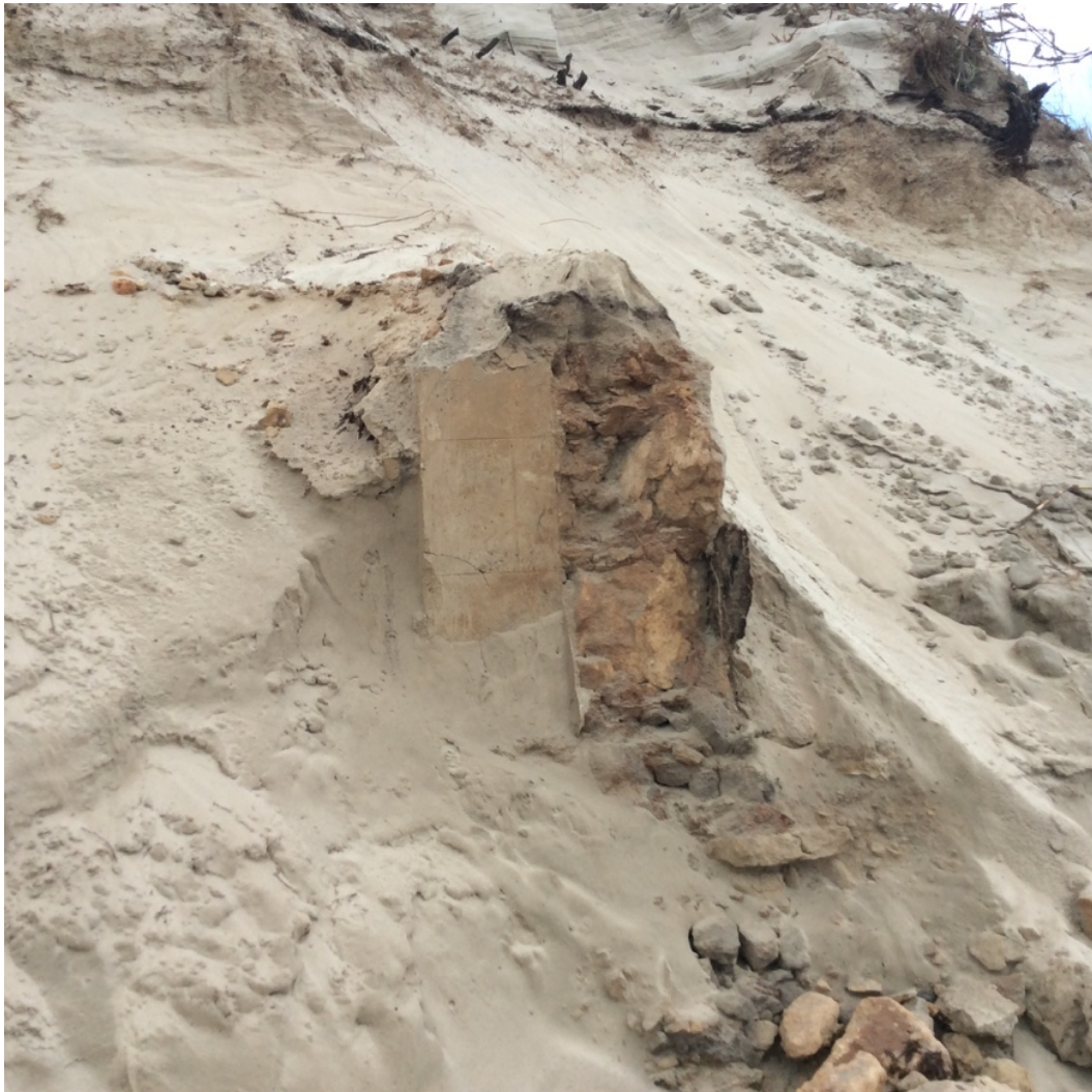
Figure 1 Stone wall exposed in foredune following storms in May 2018. Note render with tuck-pointing on front edge (Greg Horsman)
