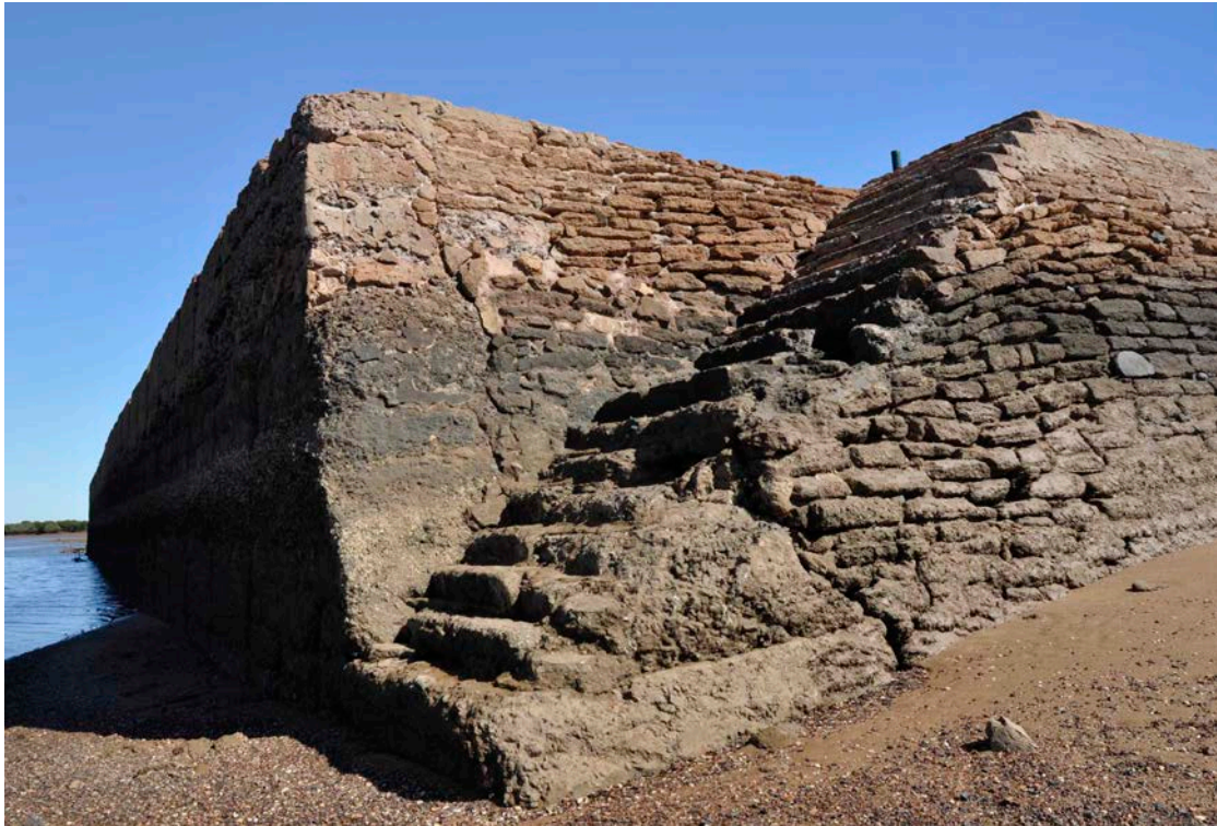
Figure 18. Steps on northern side of Cossack quay at low tide in 2012.
