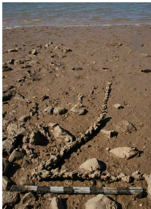
Figure 29. Corroded mooring chains are evident along the length of Butcher Inlet foreshore.
