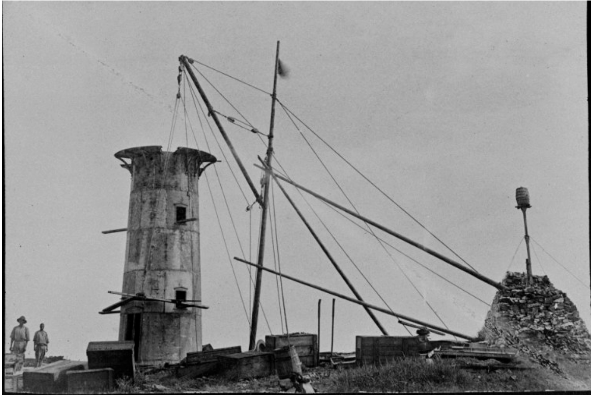
Figure 36. Jarman Island lighthouse under construction in 1887, with original tub beacon and rock cairn at right (SLWA 020827PD).
