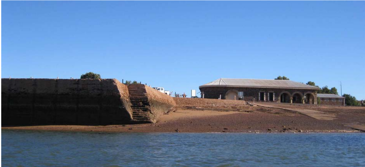
Figure 16. Cossack quay at low tide with Customs Bond Store in background and more recent concrete boat ramp. The turtle pen and swimming baths were in this area north of the quay, in front of the Customs Bond Store.
