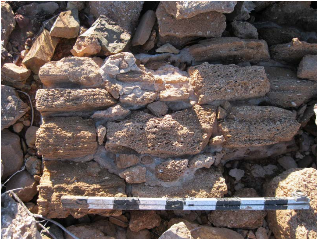
Figure 20. Mortar repair on Cossack dry stone retaining wall/ seawall.
