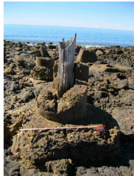
Figure 26. Point Samson jetty piles in inter-tidal zone, June 2012.
