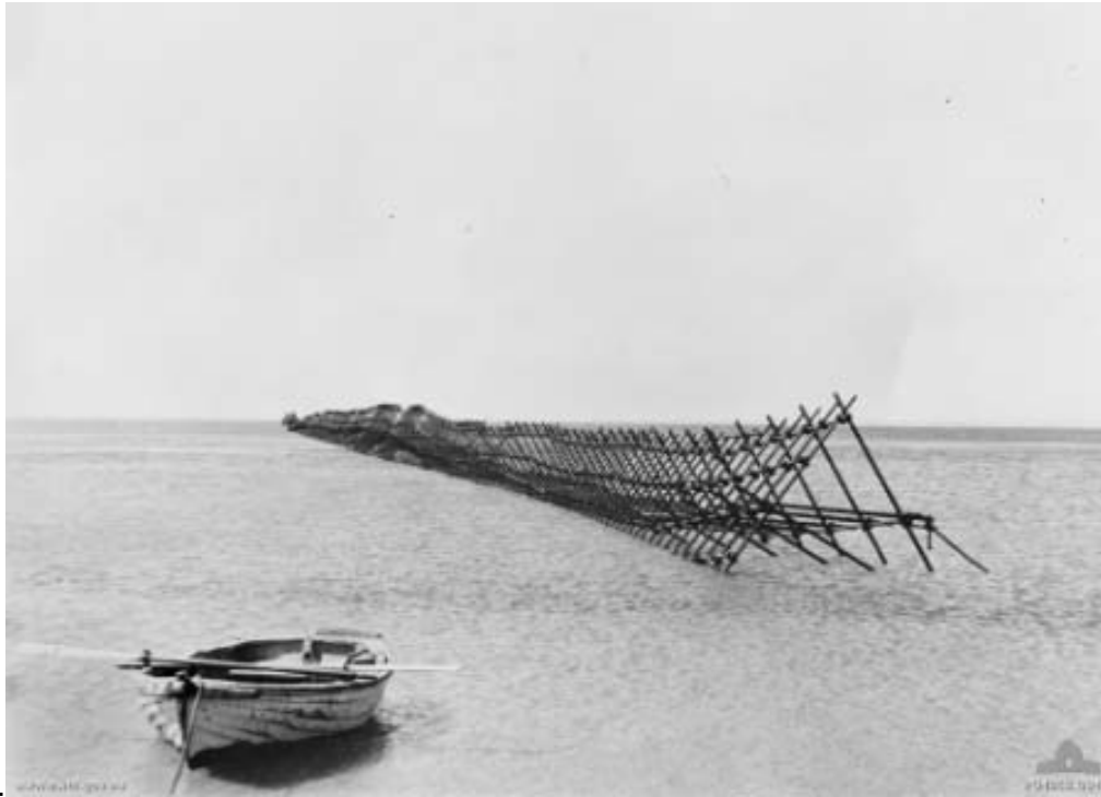
Figure 5: Type 'A' anti-boat scaffolding in Cockburn Sound (Australian War Memorial P04262.004)
