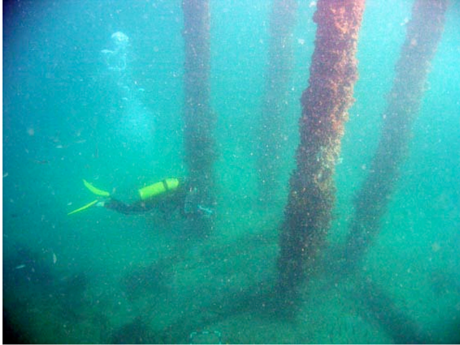
Figure 7: Diver and piles of Dolphin No.60 underwater in April 2007. Note collapsed timber beams and piles on seabed (Patrick Baker/ WA Museum)
