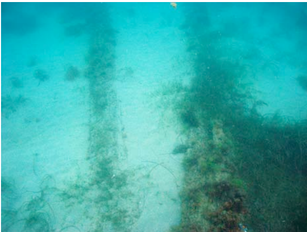
Figures 18 and 19: Two large timber piles from a collapsed intermediate support four pile dolphin, with detail of cross head timber bracing at ASN005. (Jeremy Green/ WA Museum)
