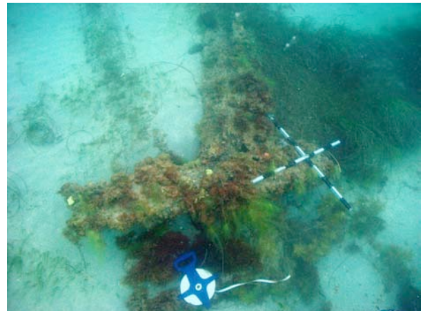
Figures 18 and 19: Two large timber piles from a collapsed intermediate support four pile dolphin, with detail of cross head timber bracing at ASN005. (Jeremy Green/ WA Museum)
