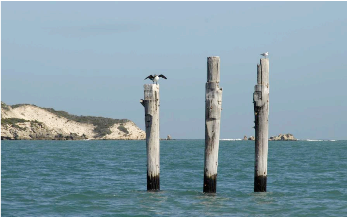
Figure 9: Dolphin No.60 structure in May 2008 after collapse of southeast pile, view looking west. (Patrick Baker/ WA Museum)
