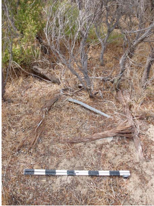
Figure 24: Corroding steel anti-submarine net cable at Woodman Point in February 2010. (Matt Carter/ WA Museum)
