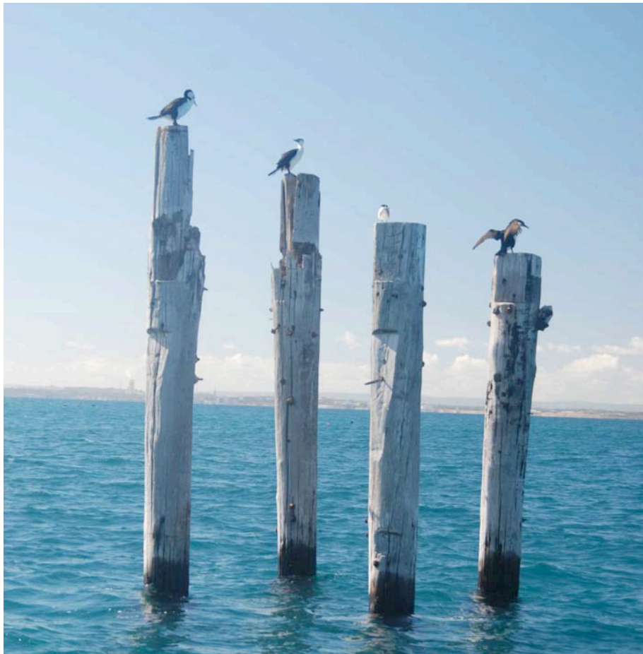
Figure 6: Timber pile structure off Garden Island since identified as Dolphin No. 60 in April 2007 after loss of timber platform bracing in a storm in 2006, view looking southeast. (Patrick Baker/ WA Museum)
