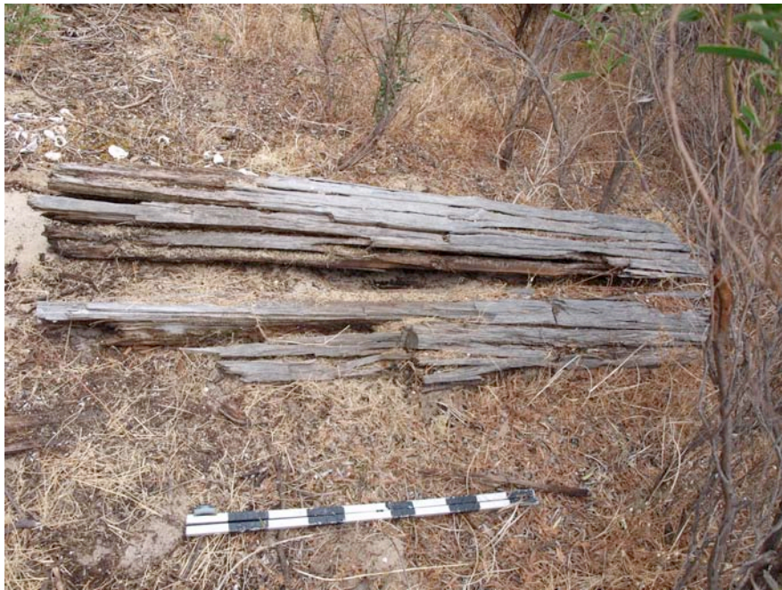
Figure 25: Deteriorated remains of anti-submarine defence timber pile at Woodman Point in February 2010. (Matt Carter/ WA Museum)
