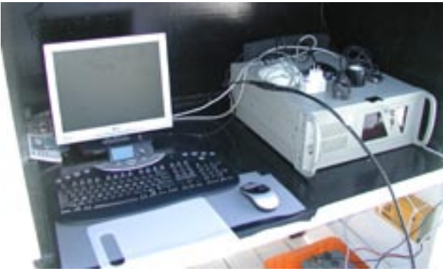
Figure 19. Close up of operations booth.
