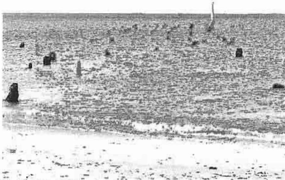
Figure 3: The Long Jetty piles
