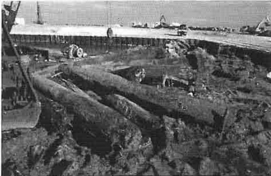
Figure 8: South Jetty piles after excavation
