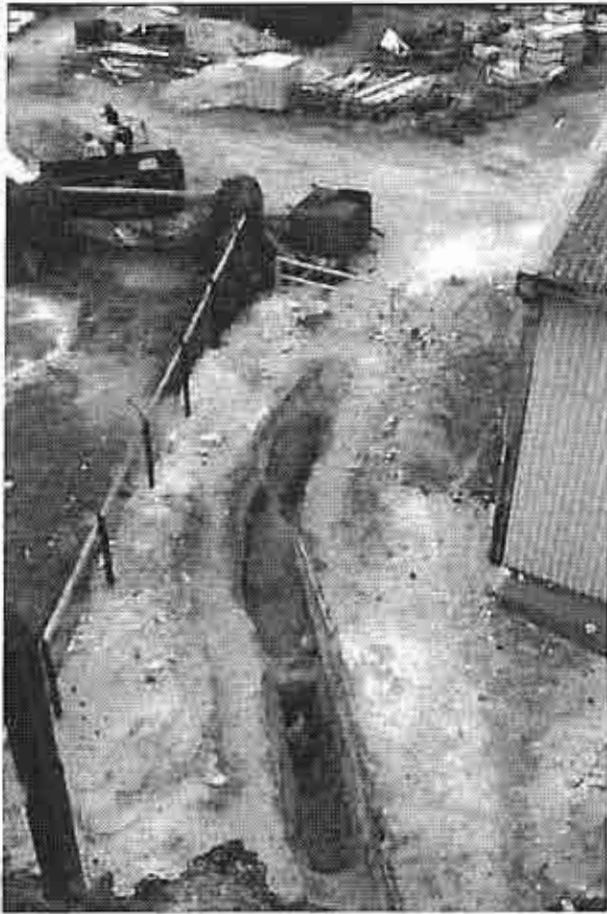
Figure 13: Bathers bay Excavation 1984. Trench at mouth of Whaler's Tunnel
