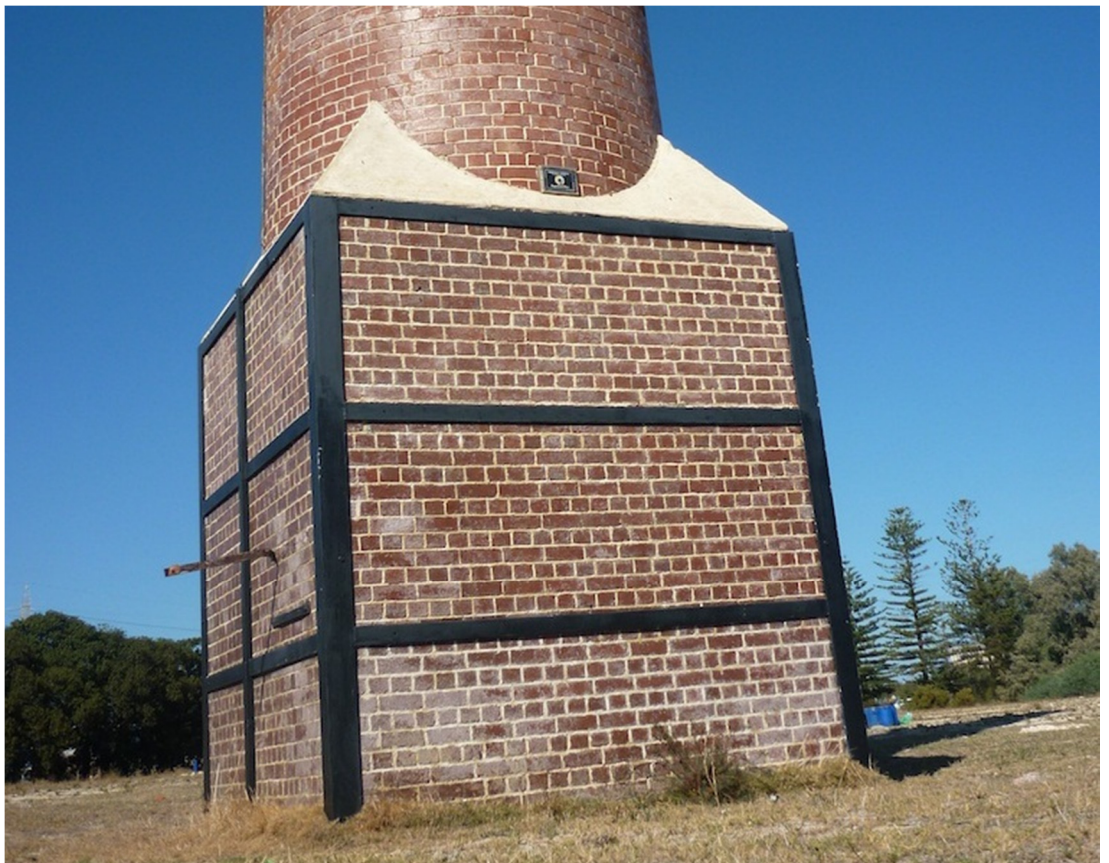
Figure 4-12 Base of Robb Jetty Abattoir chimney (Danielle Wilkinson, May 13, 2011).
