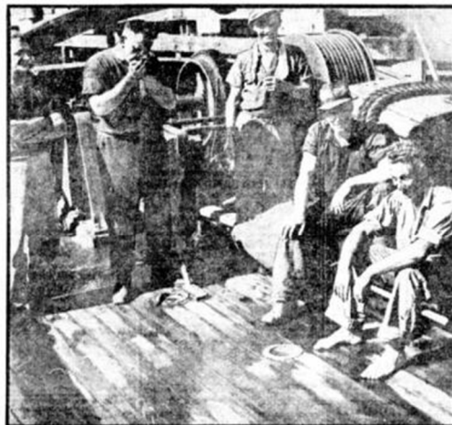
• Wyola's crew has a smoke-a between jobs. Work starts in the early hours of the morning, often finishes late at night. Crew make up in time off or overtime. Fireman Joe Rowe has been in Wyola for 13 years, was once machine-miner on goldfields.
