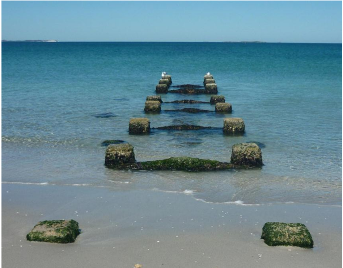
Figure 4-13 Shallow section of Robb Jetty remains, with effluent pipe running along the middle of the piles (Danielle Wilkinson, October 26, 2012).
