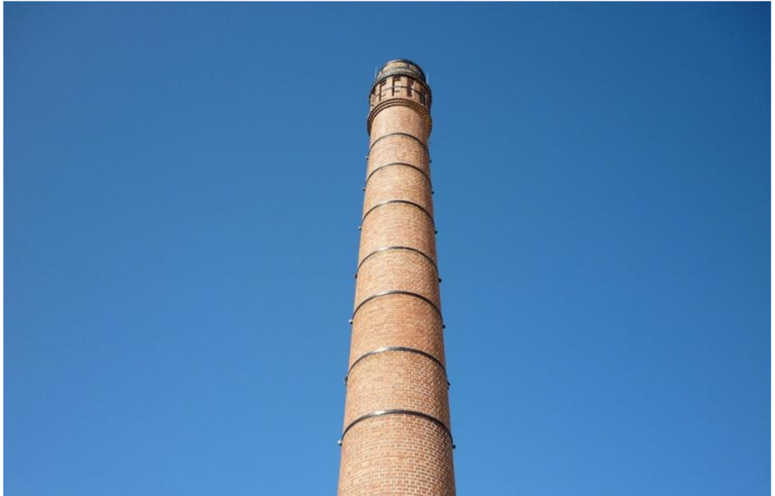
Figure 4-11 Stack of Robb Jetty Abattoir chimney (Danielle Wilkinson, May 13, 2011).
