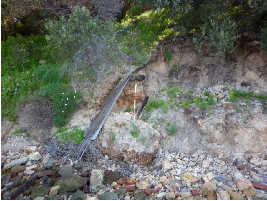
Figure 56: Timber planking of Mt Lyell Stairs
