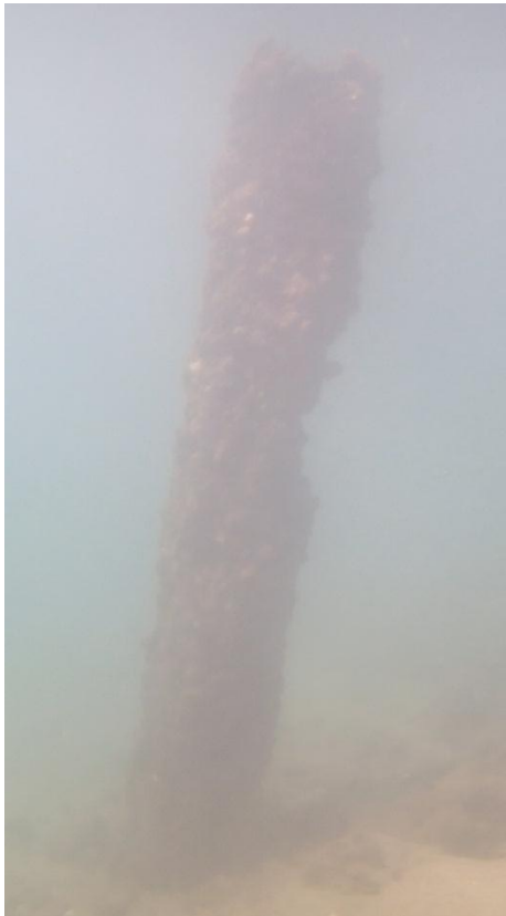
Figure 19: Remains of pile adjacent City of Perth
