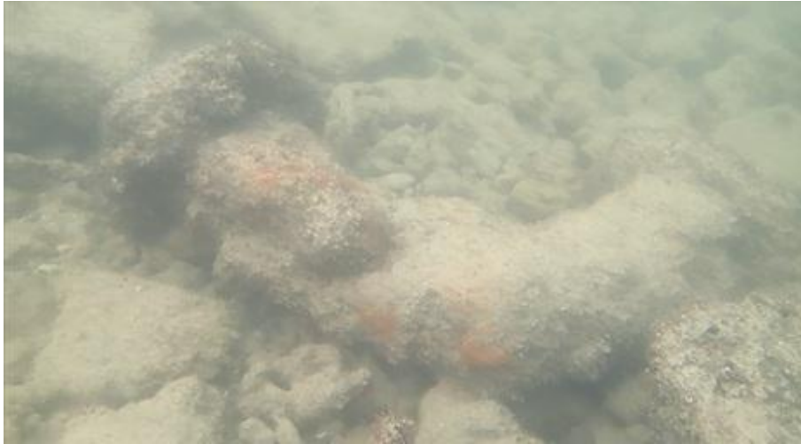
Figure 48: 90 Degree pipe angle with intact flanges
