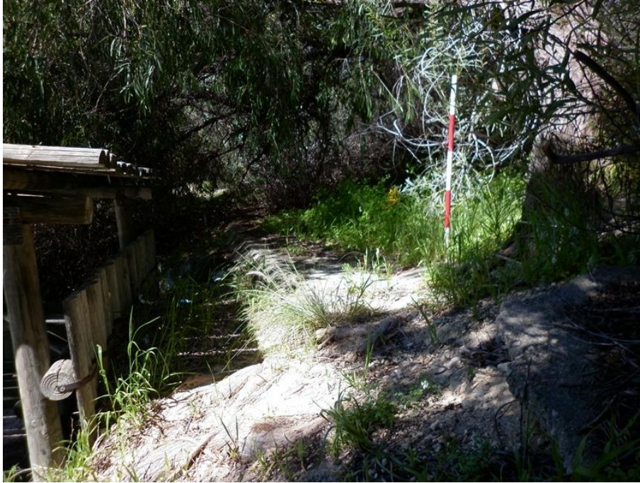
Figure 80: Old road surface, Pt. Direction.
