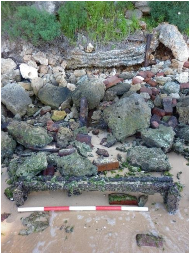
Figure 57: Railway track step at Mt Lyell Stairs
