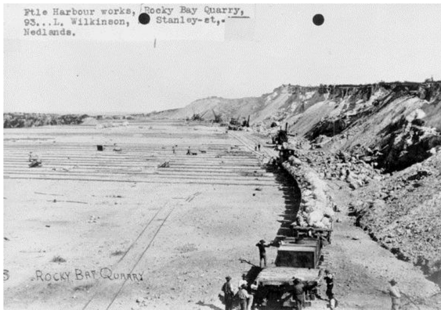
Figure 9: Looking West across the level limestone platform resulting from quarrying, Rocky Bay. Rail was one method of transporting the limestone blocks to the work area (Source Battye Library Online Collection 3045B22)
