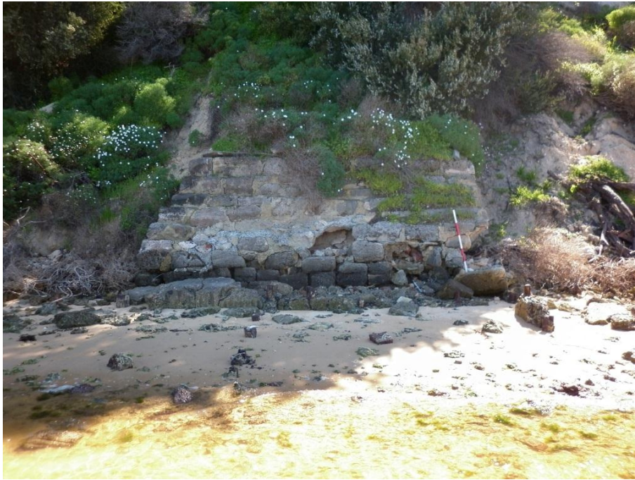
Figure 51: Limestone wall of Mt Lyell Jetty
