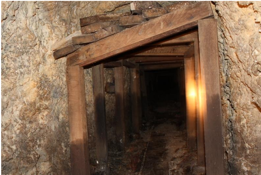
Figure 75: Wooden shoring within the soap factory tunnel
