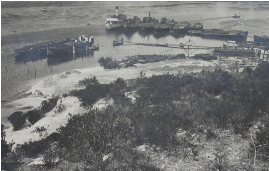
Figure 8: Remains of Point Direction barges destroyed during slipway construction, 10th March 1943 (Source: Kenny n.d.)
