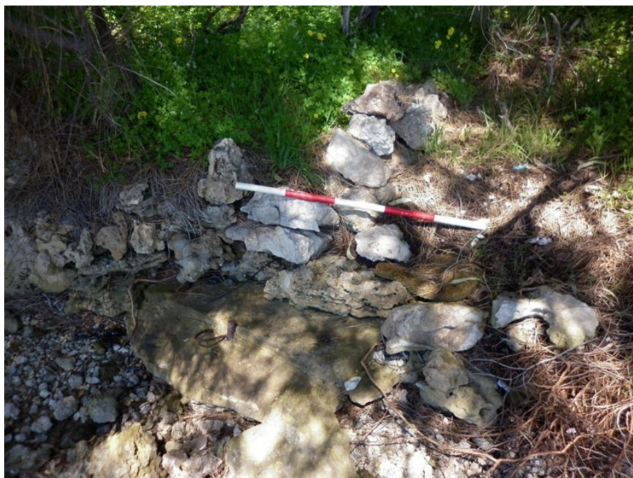
Figure 79: Concrete foundation set with metal ring and pipe base. Note the dry stone wall built on top of the foundation.
