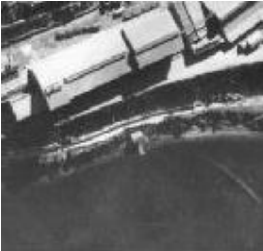
Figure 44: 1959 image of Mt Lyell Pumping Station (WA 534 Z Metro Regional Run 26 (39-79) 3750' 6" Jun 1959 26/77)
