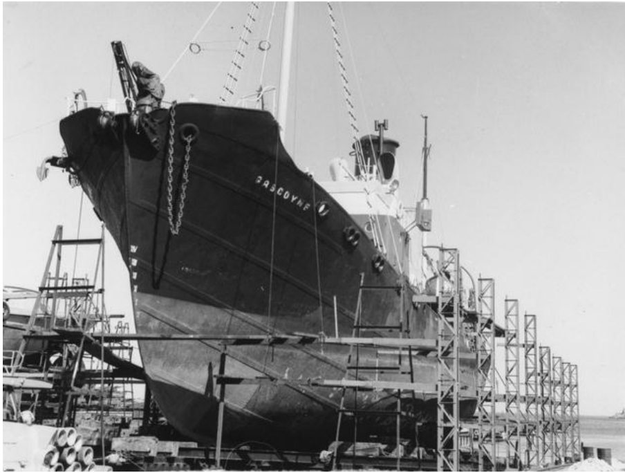
Figure 82: Whale chaser SS Gascoyne on slipway in 1962 (Source: WAMM D7/430b)
