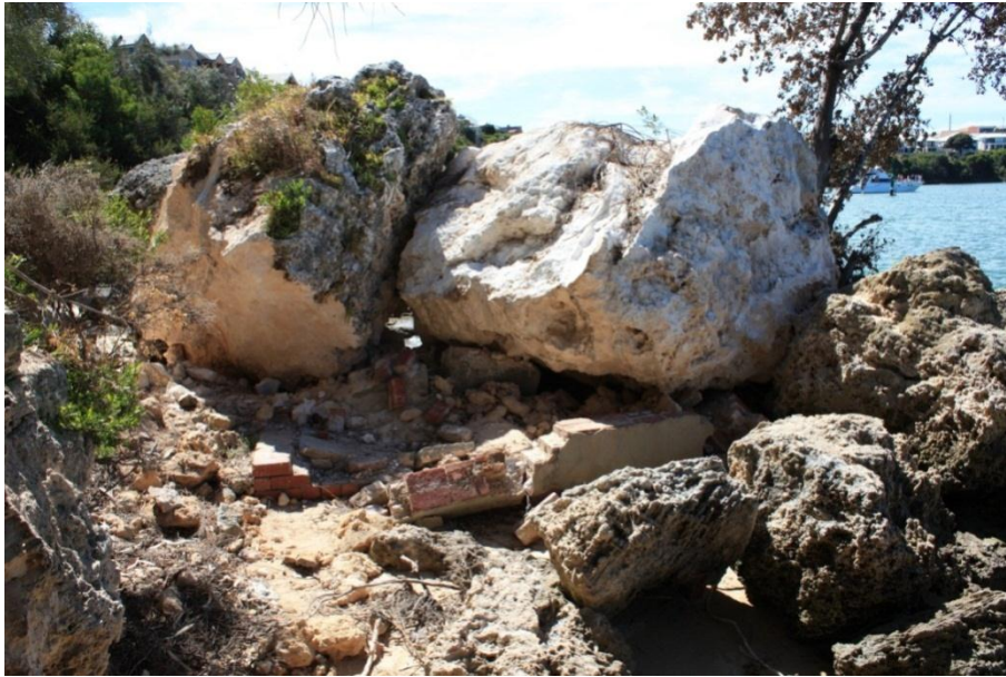
Figure 12: Rockfall onto pump house foundations
