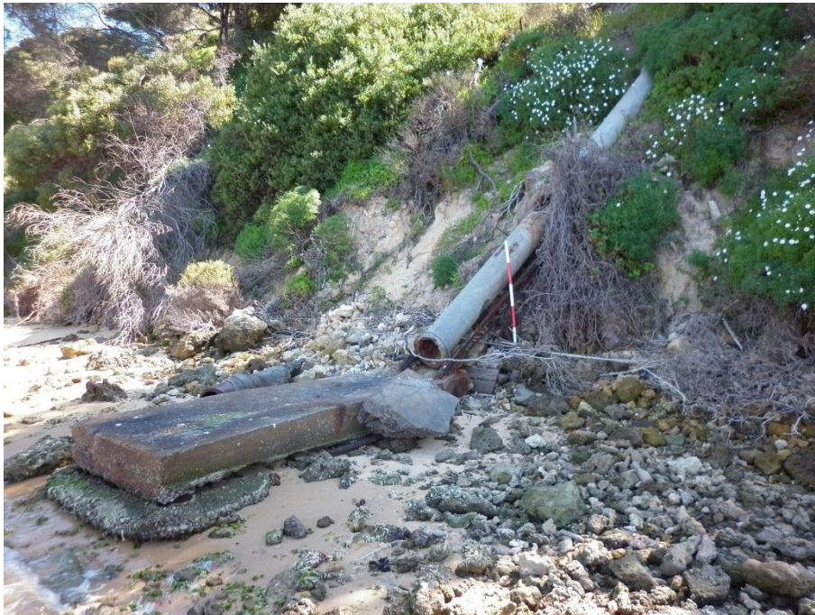
Figure 54: Drain west of Mt Lyell Jetty
