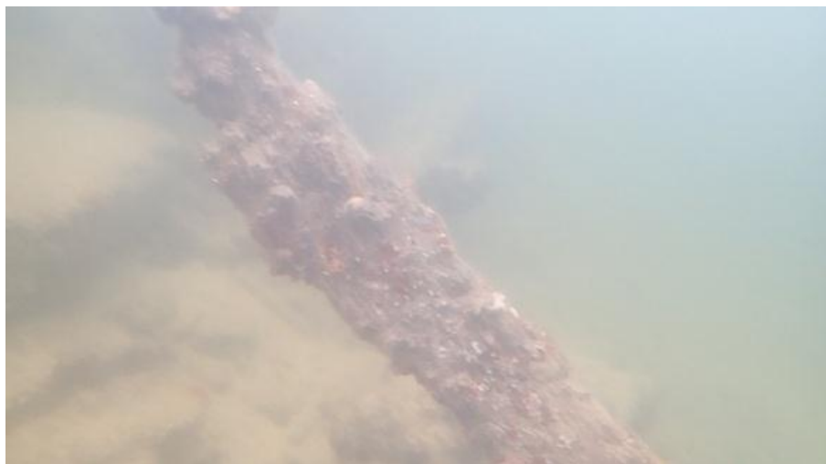
Figure 47: Example of structural iron present on site
