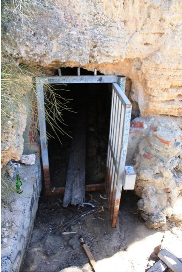
Figure 74: Entrance to the soap factory tunnel.
