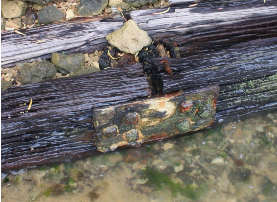
Figure 61: Fastening plate typical of all timber joins in the slipway
