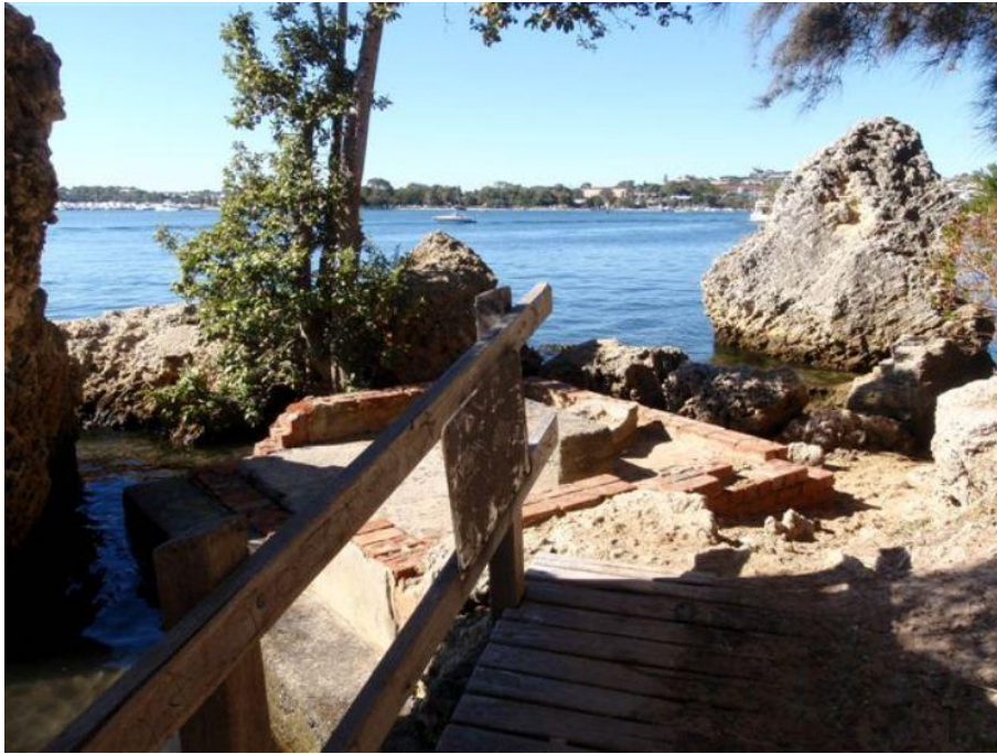
Figure 68: Concrete platform associated with the soap factory pump house, June 2009
