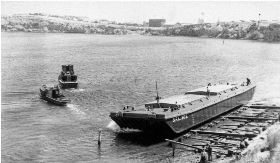
Figure 7: Steel Barge SPL302 being launched ca.1942 (Source WAMM: MHA / 4577 / 23)
