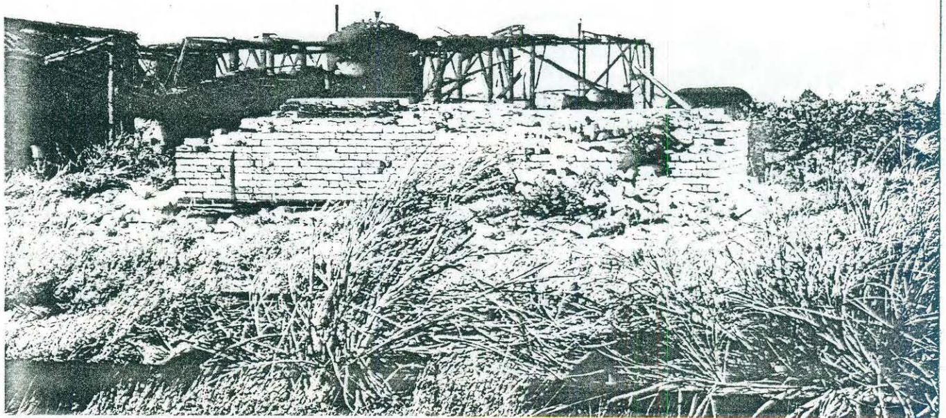
Fig. 21. Brick firebox from the south.
